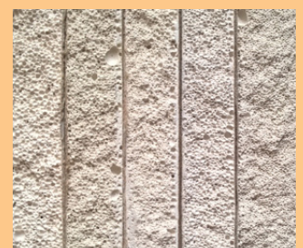
Different bubble structures of gypsum wallboards
